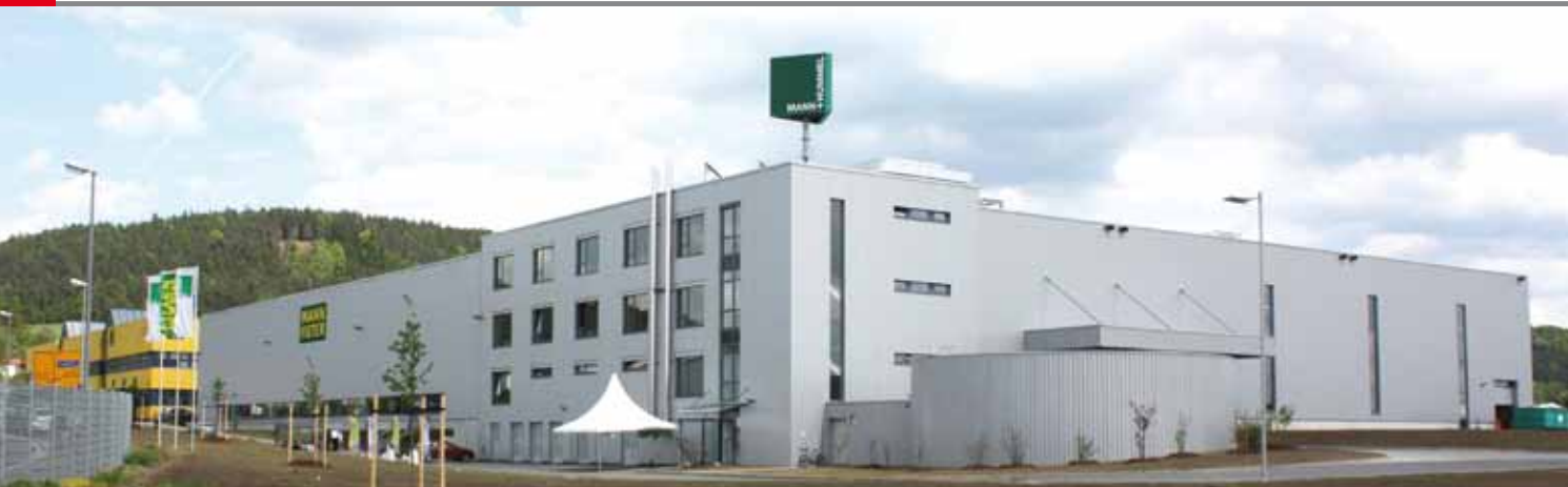
MANN+HUMMEL's new plant for cabin air filters in Himmelkron
